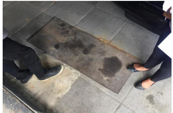
BAK SEPTIC TANK
