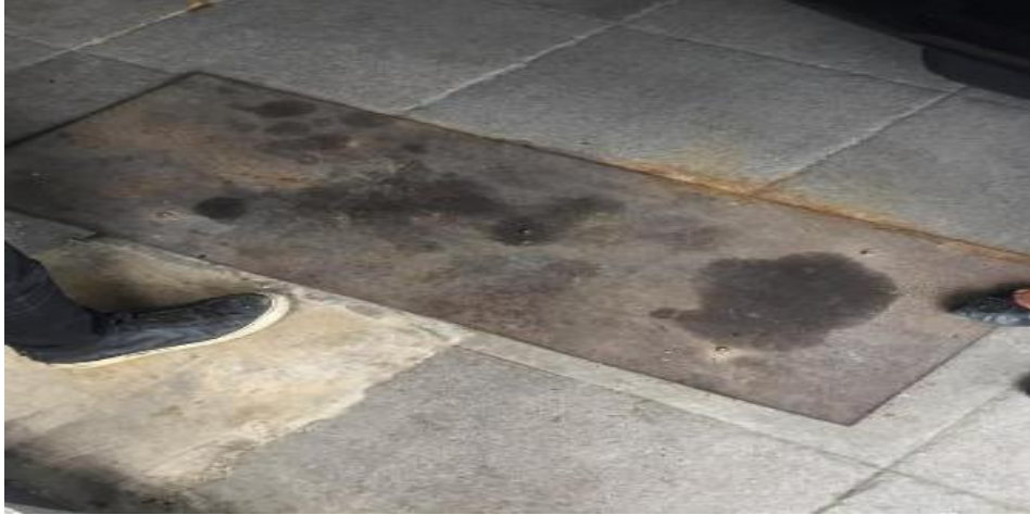
Gambar 4. 2 Bak Septic Tank
